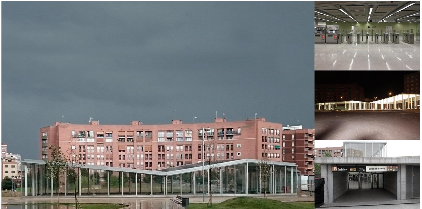
new hall and platform accesses
